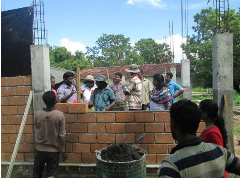
New community centre under construction with Mud Concrete Blocks.
