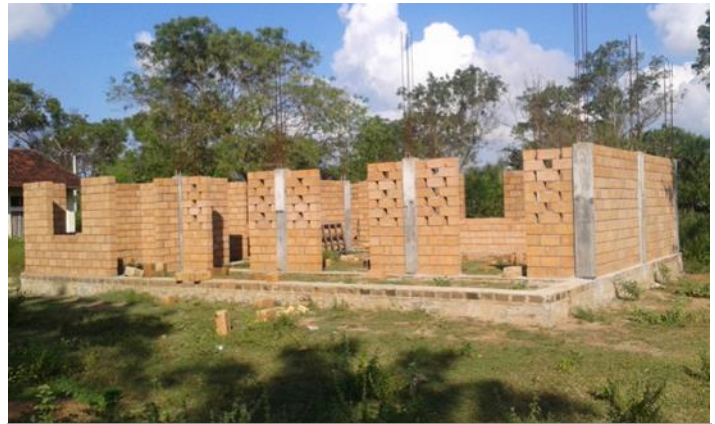
Construction work at lintel level.
