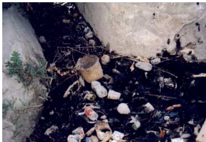
Photo 3: Open sewer in Caicoli
