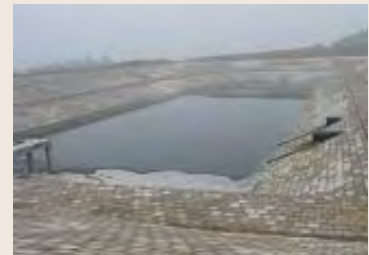
Fukuoka Method leachate collection pond in Weifang City, China.
